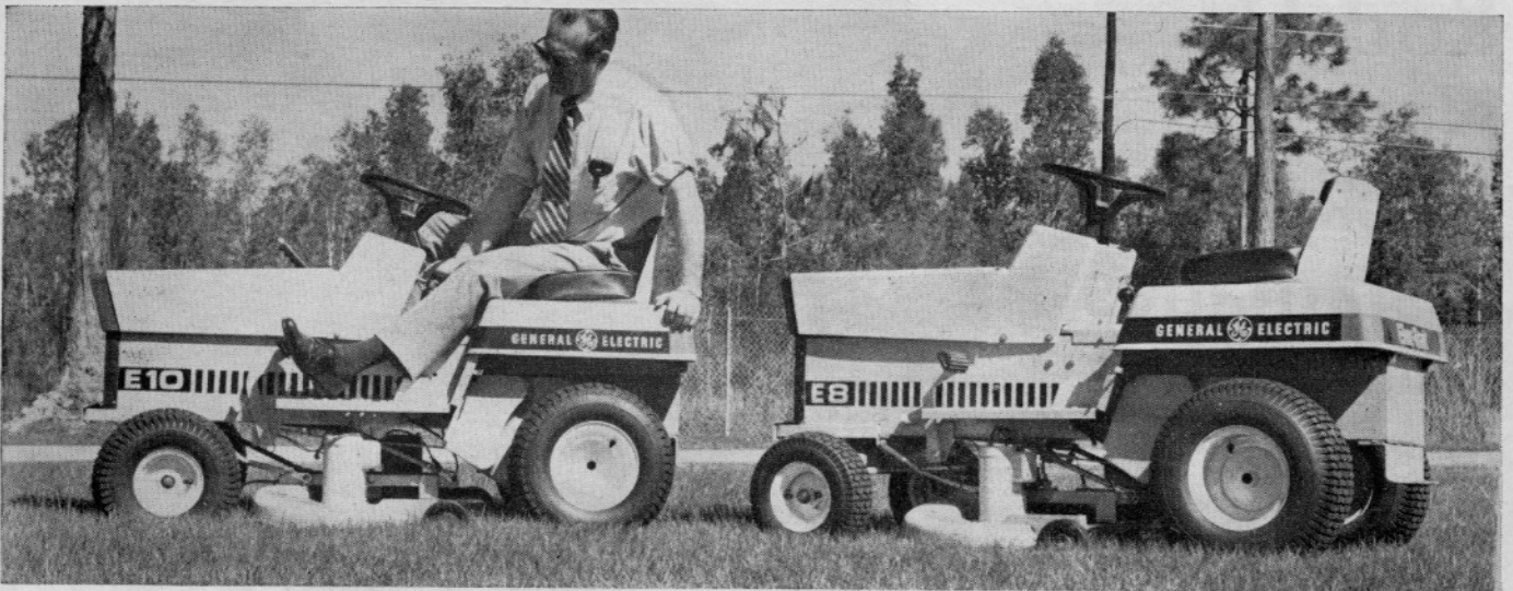
Ten and eight-hp Electraks look alike, but E-10 has extra batteries. The E-8 will cut an acre per charge, E-10 one to three acres.
