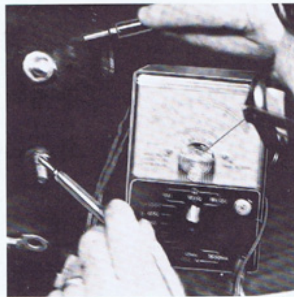
22. Multitester set on RX10 wires disconnected from motor. One probe placed on motor armature stud, the other probe placed on scratched portion of the motor case. Approximately \infty ohms reading on the multitester is normal. More than 1/2-scale deflection indicates the motor armature shorted to the case. (Picture shows short.)
